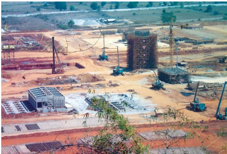
Pinpet iron factory under construction in February 2009
