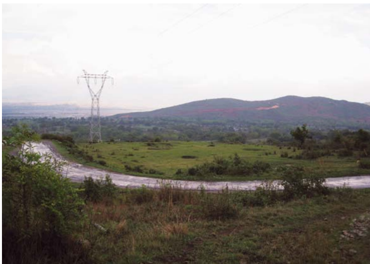
Transmission lines from Kengtawng hydropower station to Mount Pinpet. Photo taken in May 2009
