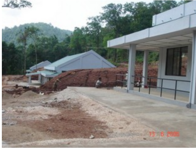
Buildings under construction at the Thabeikkyin Nuclear Battalion (DVB)
