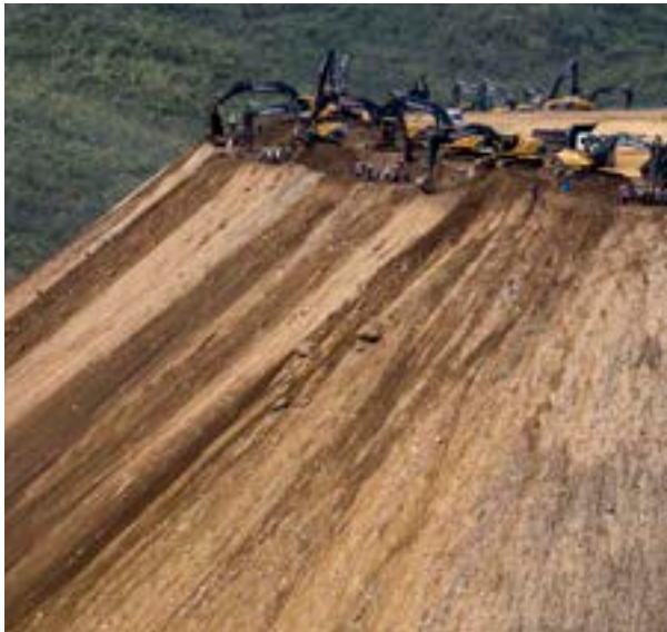
As companies ramp up mining activity, life-threatening landslides are increasingly common. At this site, at least 20 people were killed in January 2015 when heavy rains caused a waste dump collapse. CREDIT: Minzayar
