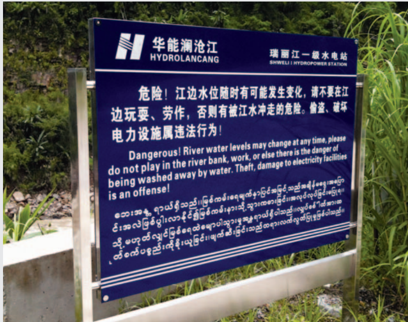
A signboard at the Shweli 1 dam warns local residents to stay away from the river bank as water levels can change at any time
