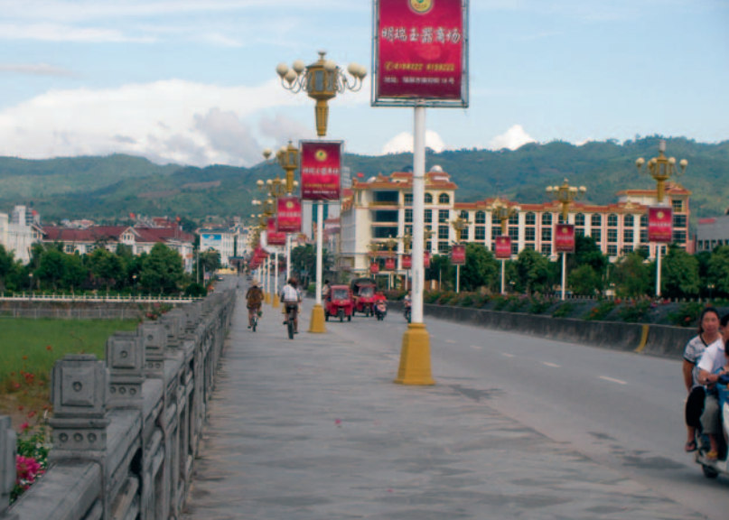
The Jegao Bridge over the Nam Mao/Shweli River
